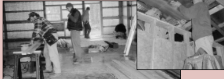
Framing New Building
